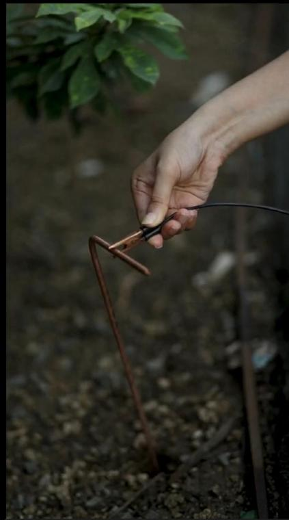
Connect the crocodile clip of the earthing wire to the earthing rod.
